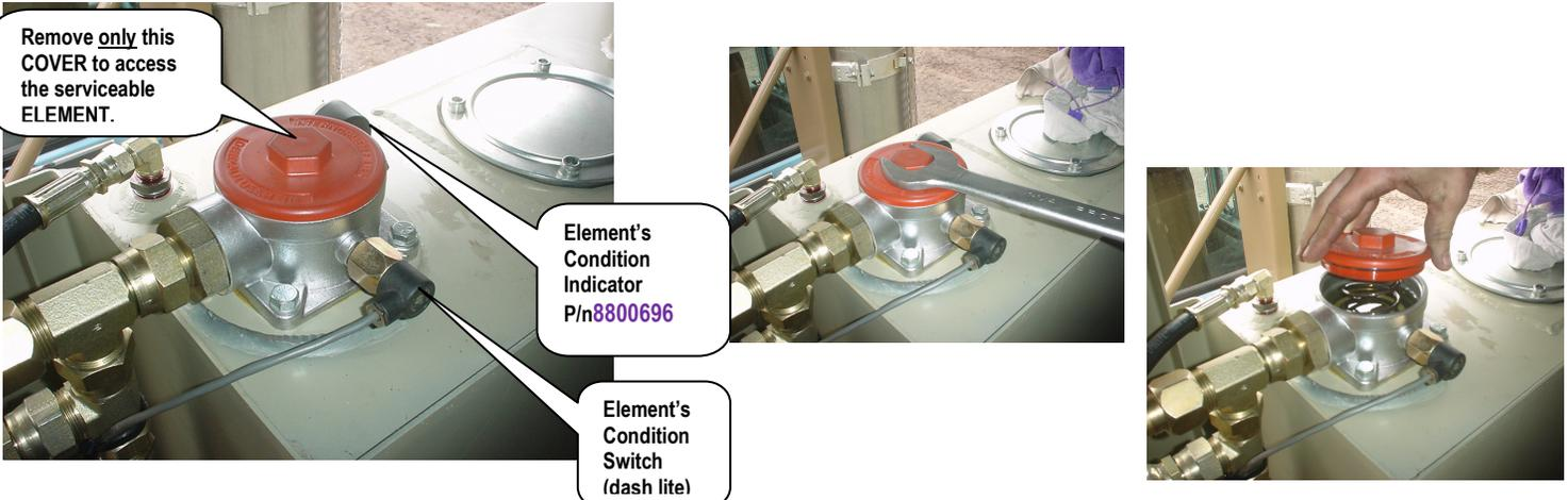
2- Remove the Filter's Top Cover by turning CCW. The Cover's compression spring will be "pushing"...so use your hand over the Red removable polymer cover when it is close to being fully un-threaded to control.
